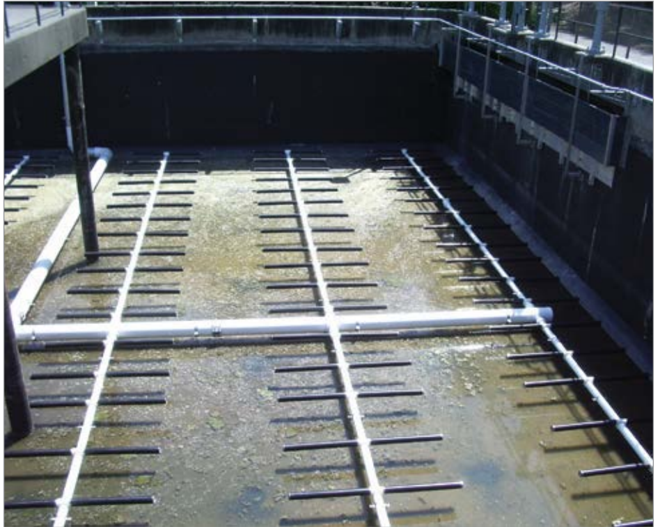
The Snappy Saddle from Stamford Scientific offers the performance equivalent of five 9-inch disc diffusers.
