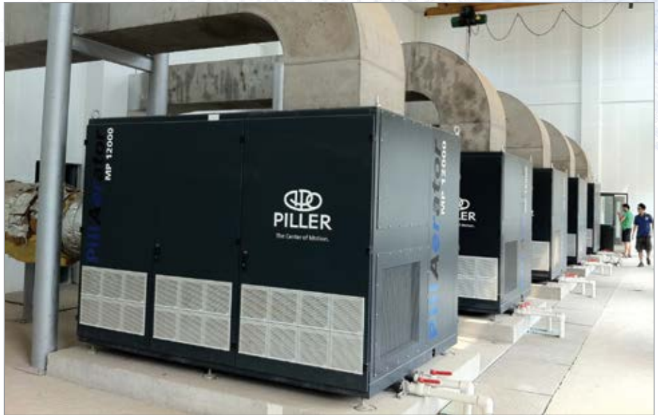
Figure 1: High-speed turbo blowers are beginning to be adopted for yeast fermentation applications, largely due to the technology's energy-saving potential.
