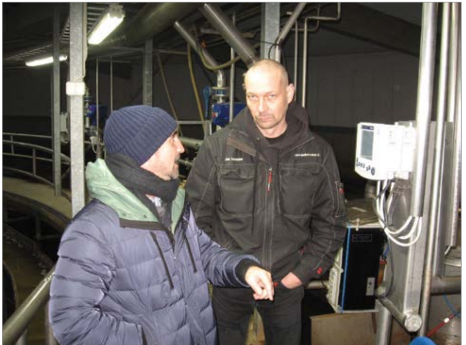
Roberto Amboldi from Stamford Scientific (left) and Jani Savolainen of Solid Water Oy (right) work to address the challenges at the Ilmajoki sewage treatment plant.
