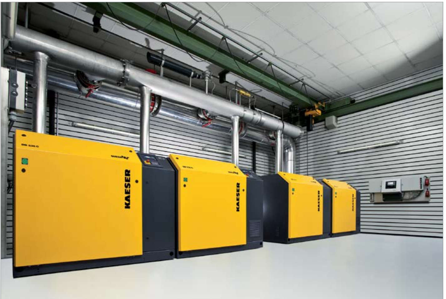
Figure 4: Multiple integrated blower packages controlled with a system master controller offer an energy-efficient and reliable solution for wastewater treatment plants.
