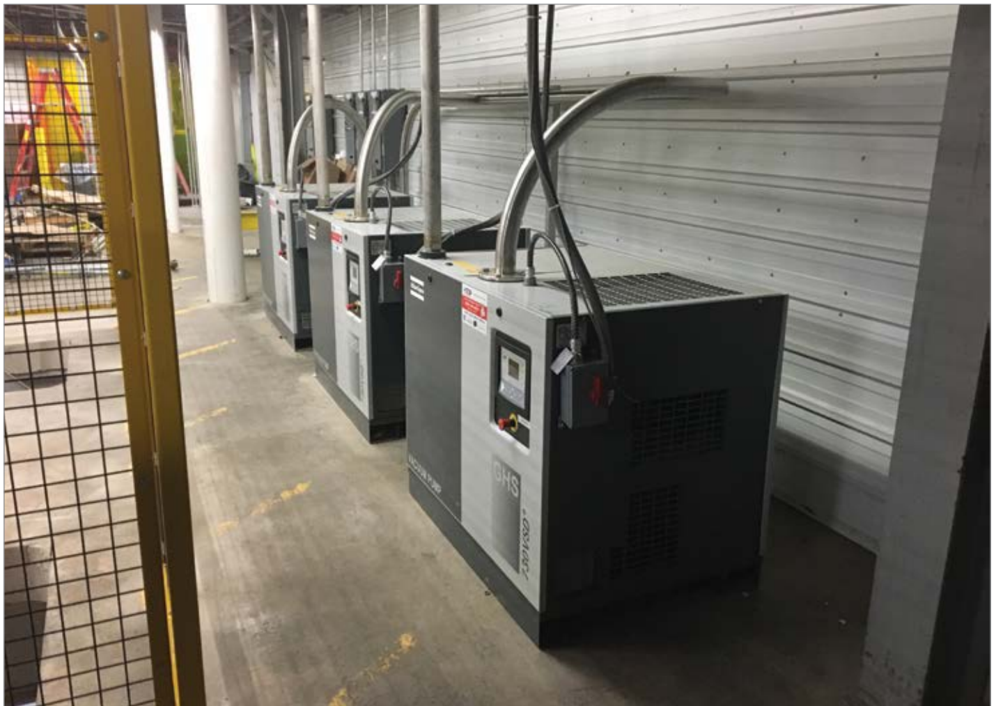
In switching to a 15 hp GHS 730 VSD+ Atlas Copco vacuum pump, customers receive more flow rate and reduce install power by 40 percent.
