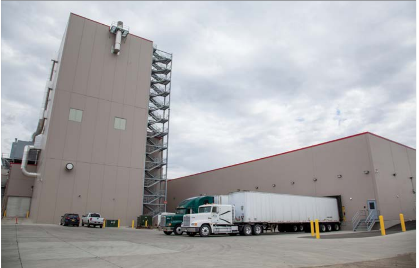
View of new dryer building at south end of plant.
