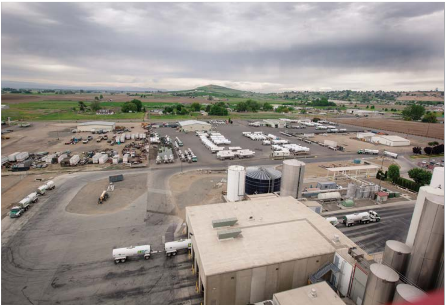
Overview of the Sunnyside plant looking towards milk receiving operation from top of dryer building.
