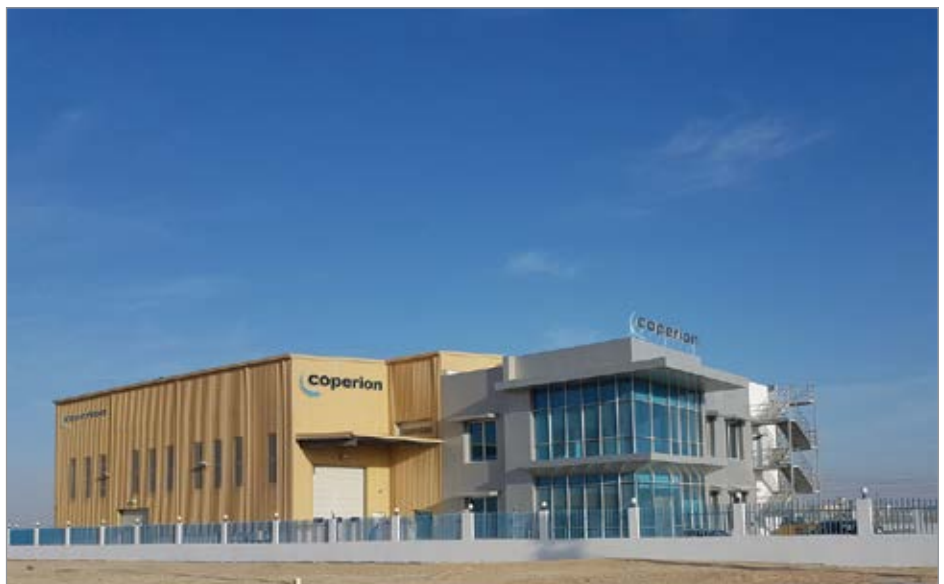
Coperion Middle East’s new facility with more than 1,400 sq. m, equipped with the most advanced machinery and a workshop tailored to deliver fast and efficient maintenance, overhaul and spare parts.
