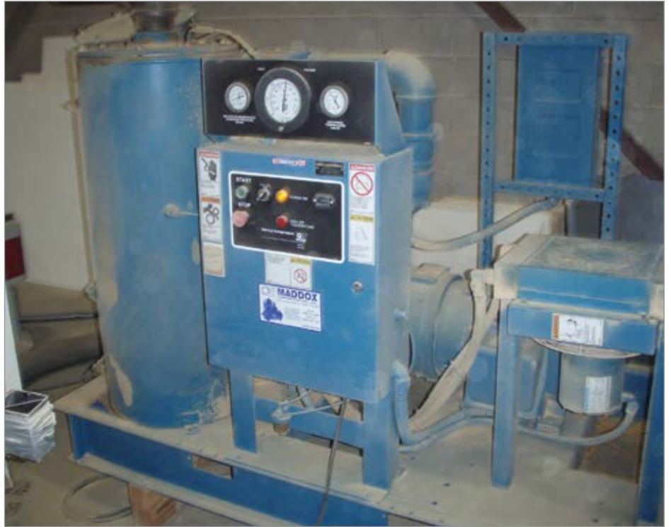
Figure 9. Typical Inlet-Modulating Rotary Screw Vacuum Pump
