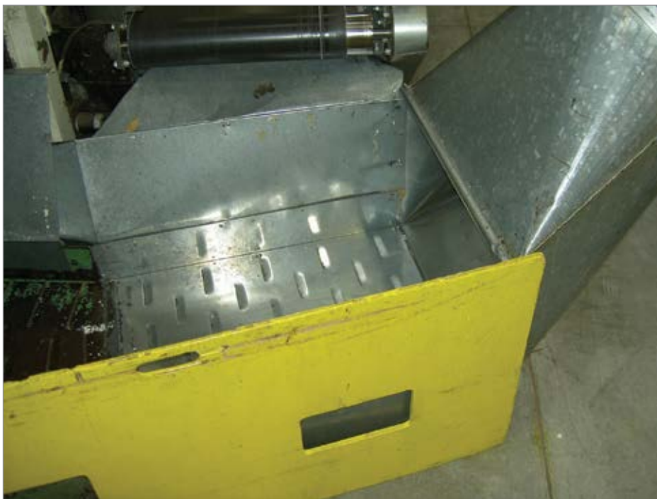
Figure 5. Typical Excessive Demand at End Use – Large Area Pick-up Point. These demands are often in trim-collection and dust-collection systems, and have high-flow and low-effectiveness due to poor design at pick-up point. Due to high-area, the velocity is not high enough at the point the material needs to be entrained in air.
