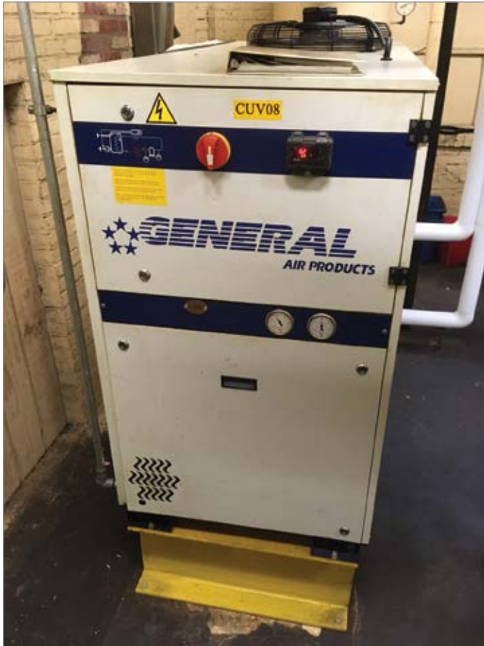
The entire cost of operating and maintaining the 16 HP (12 kW) water chiller was eliminated by upgrading to an air-cooled vacuum pump
