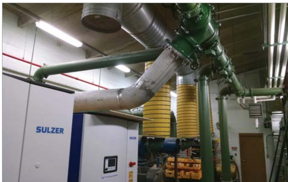
By installing Sulzer HST turbocompressors, Fraser wastewater treatment plant reduced its annual energy costs by 10%. (Photo courtesy of the Upper Fraser Valley Wastewater Treatment Plant.)
