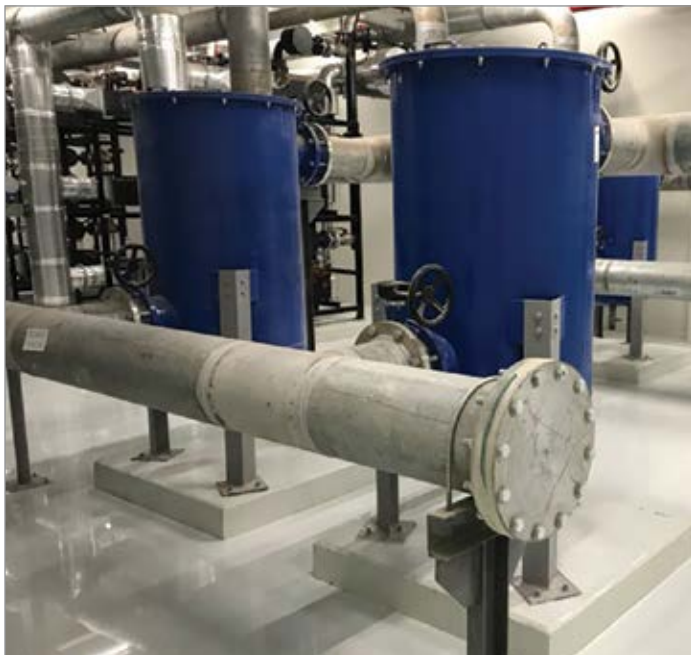
The Solberg SRS Liquid Removal System protects a vacuum pump from ingesting liquids in a vacuum drying application.
