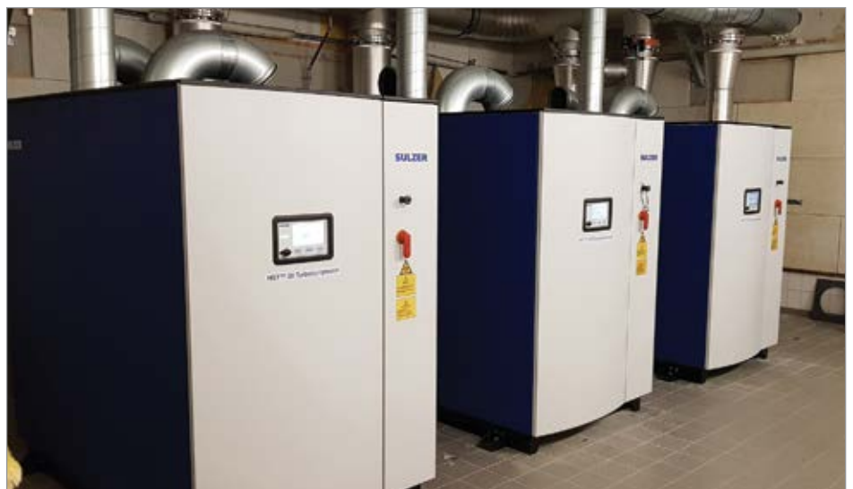
The new installation of three HST 20 units.
