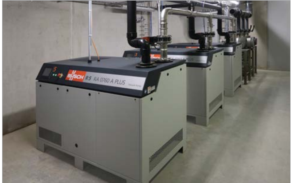
Figure 4. Modern vacuum technology with the latest PLUS Master Control unit for efficient central vacuum supply according to the actual demand.
