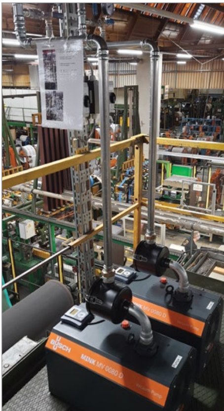
Vacuum supply with two MINK MV claw vacuum pumps for handling textile cords. Photo: Busch Vacuum Solutions
