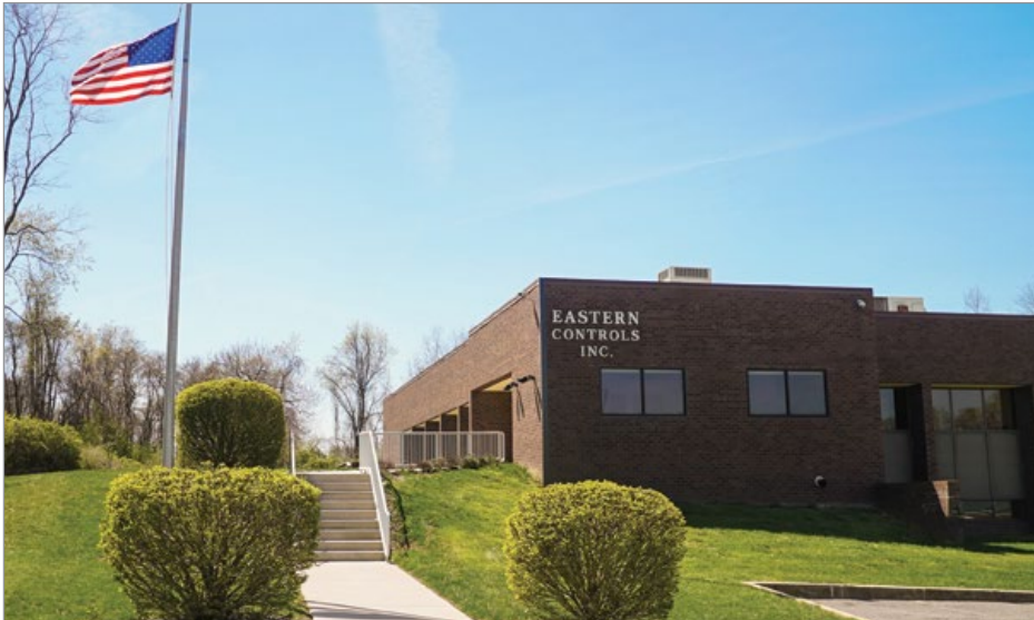
Long-time Endress+Hauser representative partner is now the exclusive authorized sales and service provider for municipalities for the east Pennsylvania, New Jersey and Delaware markets.
