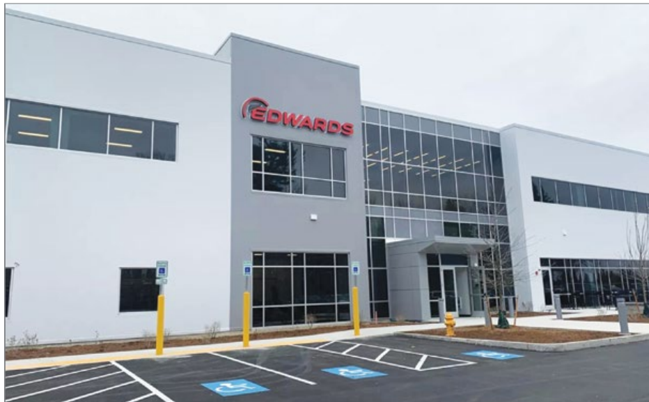
Edwards' New facility for cryopump manufacturing in Haverhill, Massachusetts.
